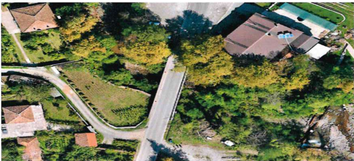
Figure 2: Klosi Bridge – Picture taken from the existing situation
