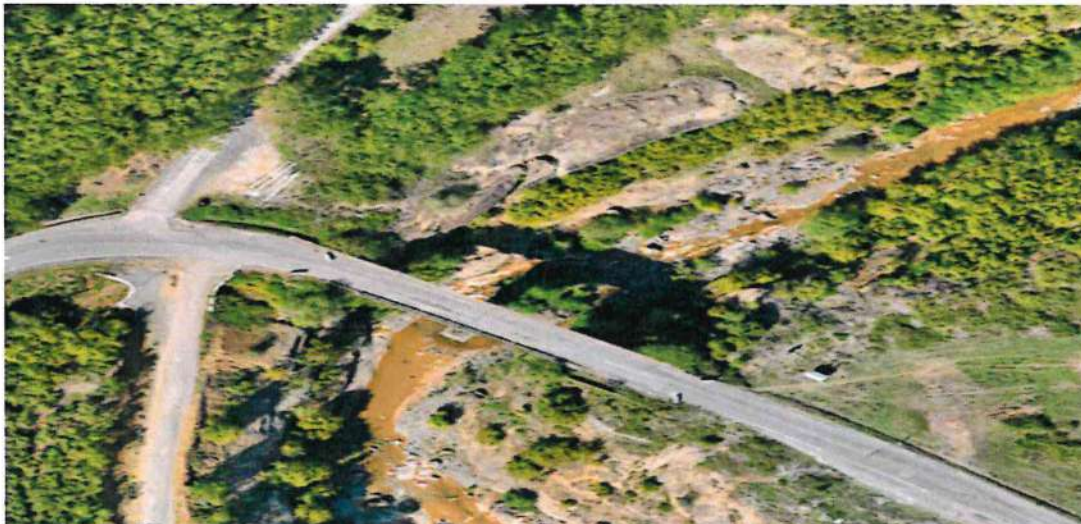
Figure 3: Karica Bridge – Picture taken from the existing situation
