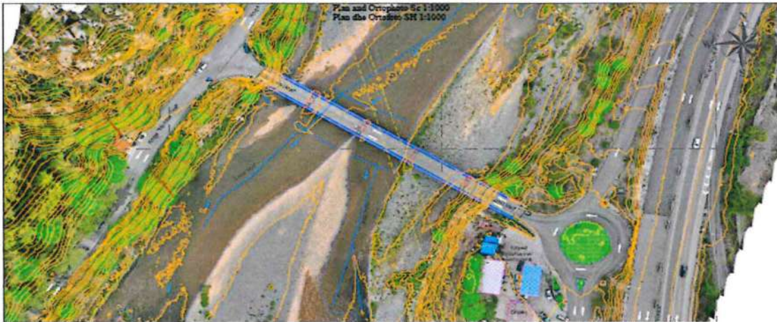
Figure 1: Uzina Rubik Bridge – Picture taken from the existing situation
